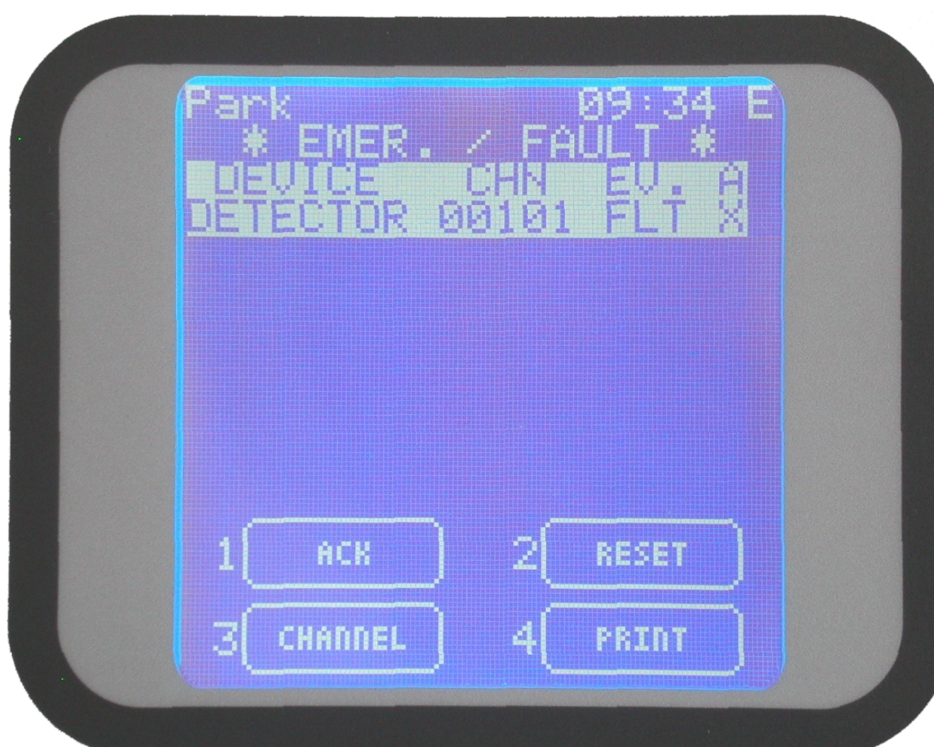
Figure 28 Active events screen with fault only
